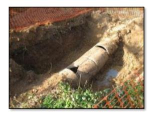
Figure 5-A damaged culvert requiring repair
