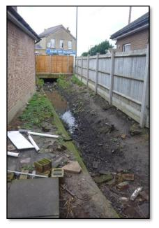
Figure 3-A ditch in need of maintenance which includes removing vegetation, silt and other debris
