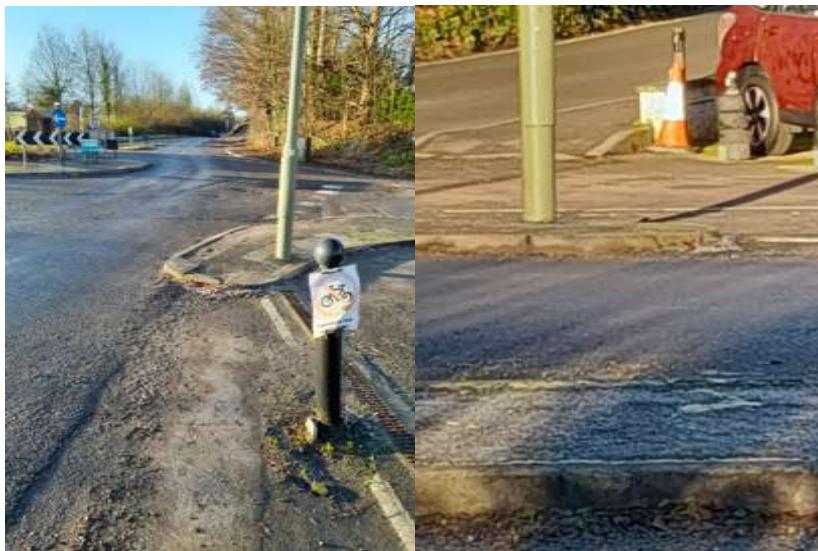
Photo 1 – no dropped curb
